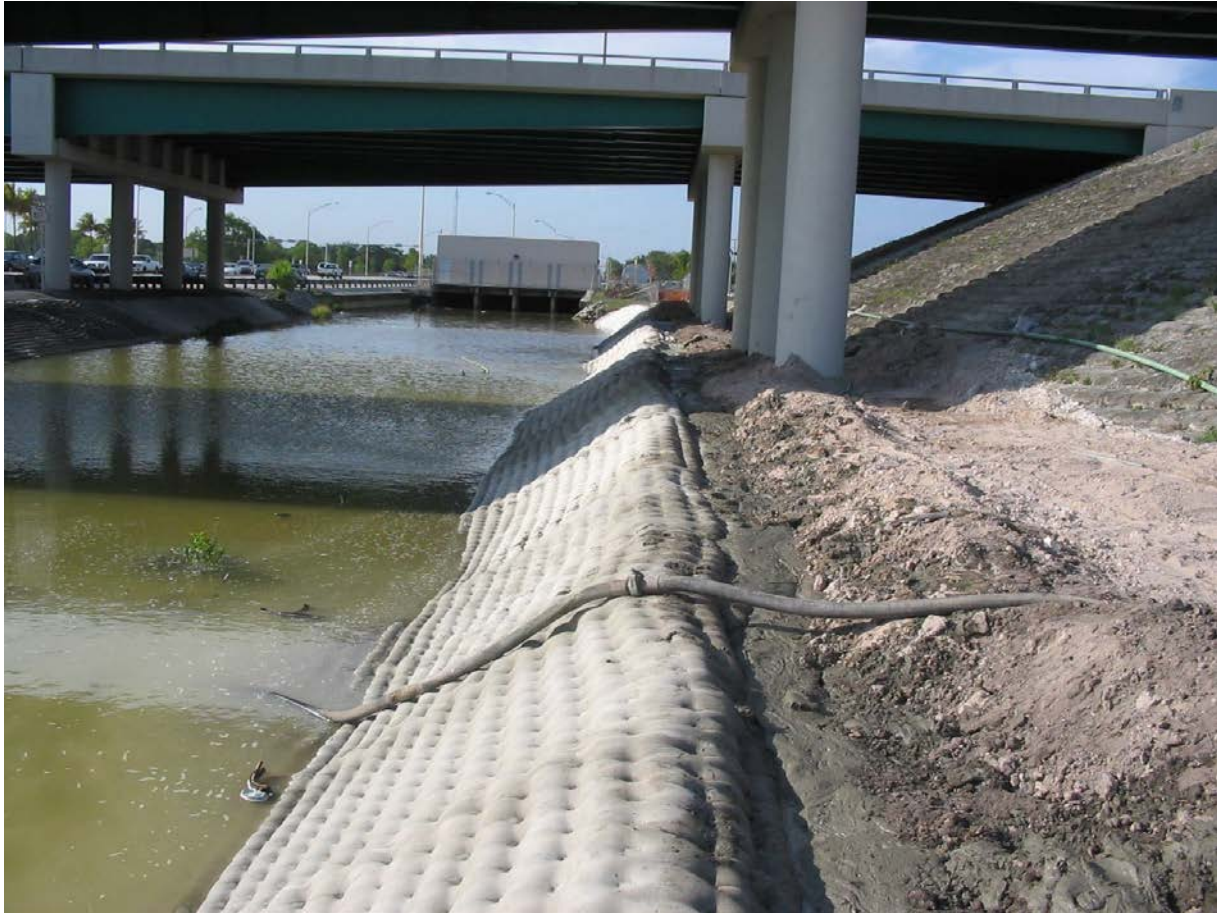
Fabric form erosion control armoring
